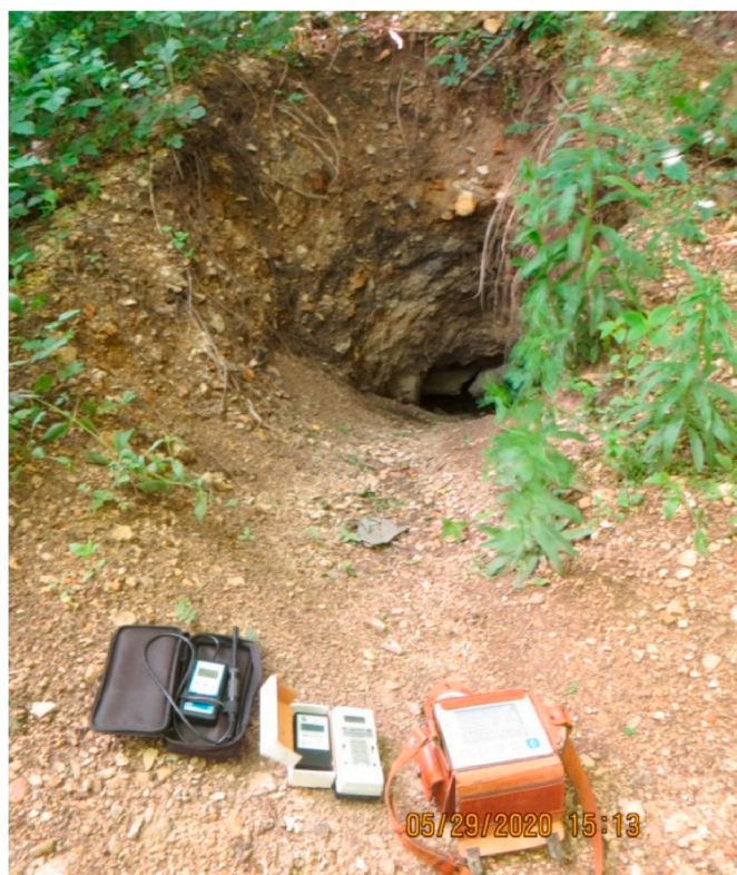
Fig. 3. A hole of likely suffusive origin above the mouth of adit #10.
